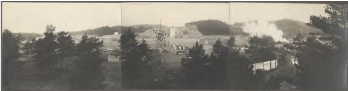
Construction of the “grand museum”, 1922. © Kröller-Müller Museum, Otterlo.
